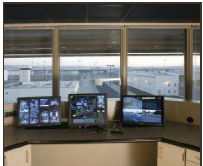
This is a view from the tower of the administration building. The center touch security monitor is flanked by split screen video monitors.
